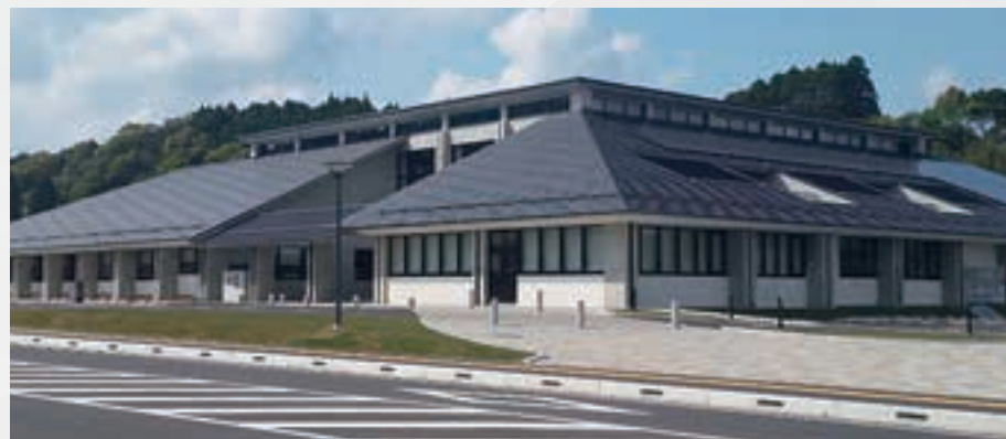
防音サッシ ※自衛隊基地周辺の防音サッシ施工例 Soundproof sashes *An example of soundproof sashes installed around a Self-Defense Forces base.
